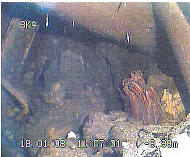
Fig. 5: Camera inspection of the exploratory drilling BK4 – broken wooden construction in a residual cavity of the former tunnel's cross section
